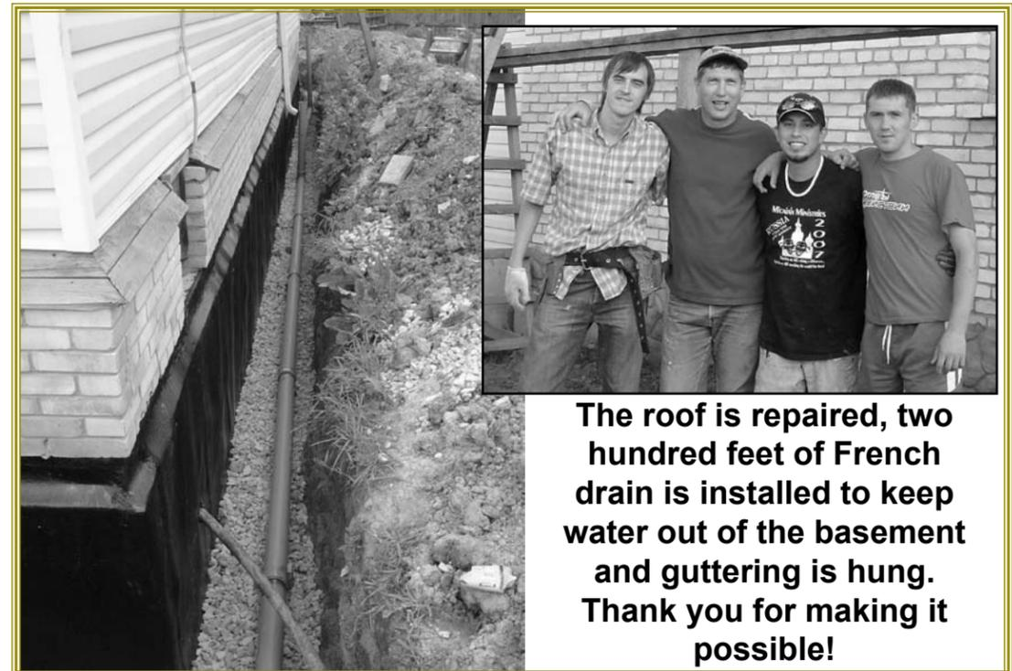
The roof is repaired, two hundred feet of French drain is installed to keep water out of the basement and guttering is hung. Thank you for making it possible!
